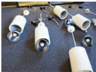
CFL downlights retrofit with Terralux LED LESENSE system, ready to be reinstalled.
